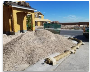
Wattles can effectively prevent discharging of landscape material.
